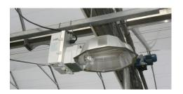
Figure 9. High Intensity Discharge (HID) luminaire in a greenhouse.
