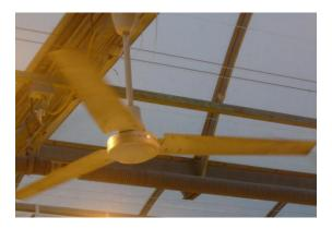
Figure 14. Paddle fan to increase vertical air movement and therefore evapotranspiration. This is important for the prevention of tipburn.
