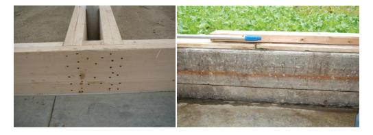
Figure 13.Edge of pond detail. The inside edges of two separate ponds made of wood and separated by structural members is shown on left. The right hand picture shows a concrete pond.
